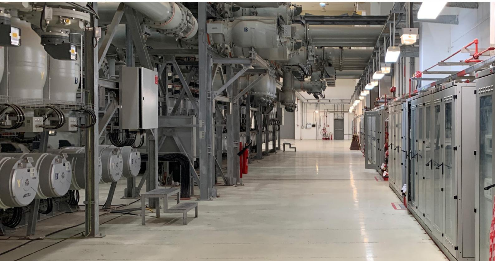
Continuous on-line PD monitoring on GIS using ultra-high frequency (UHF) measurements is an essential part of any electrical condition monitoring program to prevent unplanned outages due to defects in the insulation system of a GIS.
