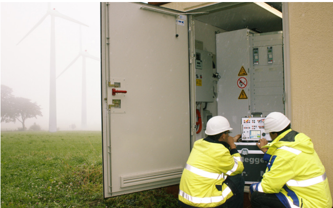
By helping detect and counteract islanding in distributed power generators, SVERKER 900's ramp instrument is useful to test frequency protection.
