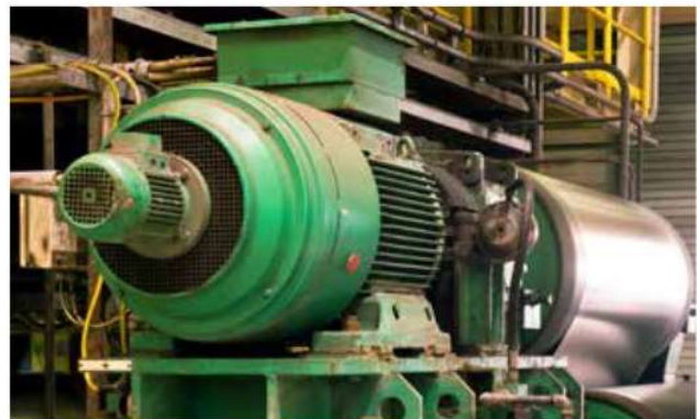
SVERKER900 eliminates concerns about test equipment power capacity and facilitates setting up the test sequence.
